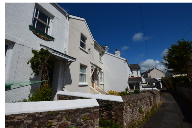
Photos of Bank End Terrace
